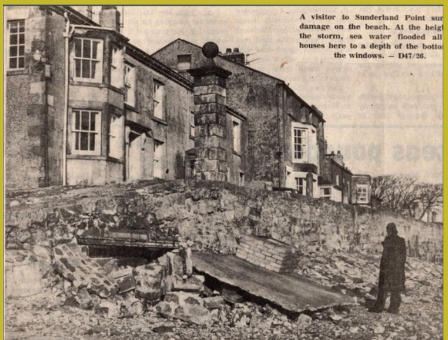
Fig. 40 Image from a newspaper article showing some of the damage of the 1977 flood. The Visitor, Flood of 1977 : Courtesy of Guardian Newspapers via sunderlandpoint.net
