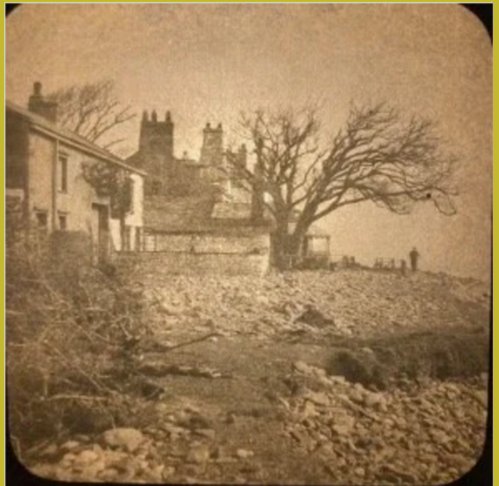
Fig. 39 Photograph of the aftermath of the flooding of 21-23 Second Terrace in 1907. Note that the area in front of the houses was grass before the flood. Gilchrist Collection.
